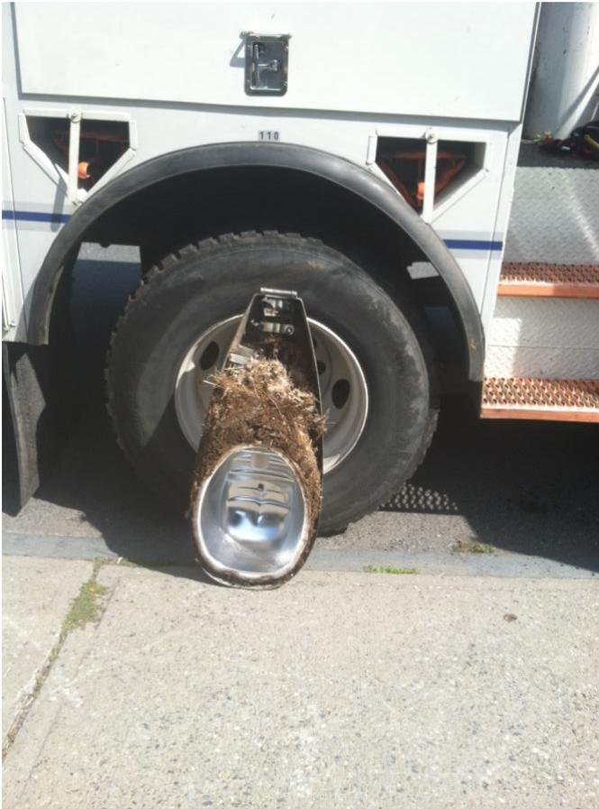
Figure 1- An HPS fixture doubling as a home for a nest on Main Street in the town of Rosendale
